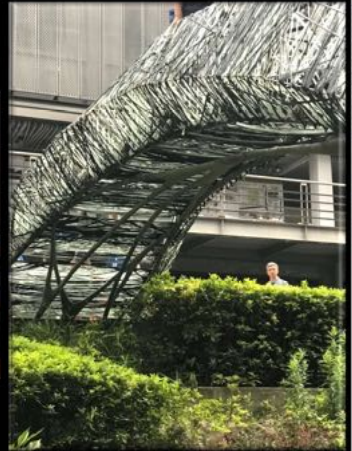
Philip Yuan's 2019 footbridge (metal printing and composite weaving) (Our BESO software, Ameba , was used for the form-finding)
